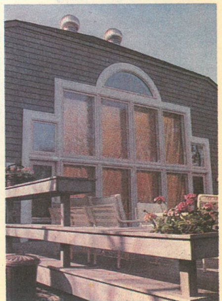
When the sun leaves the south wall, the insulating shade is lowered automatically to keep heat in the sun space for nighttime use.
