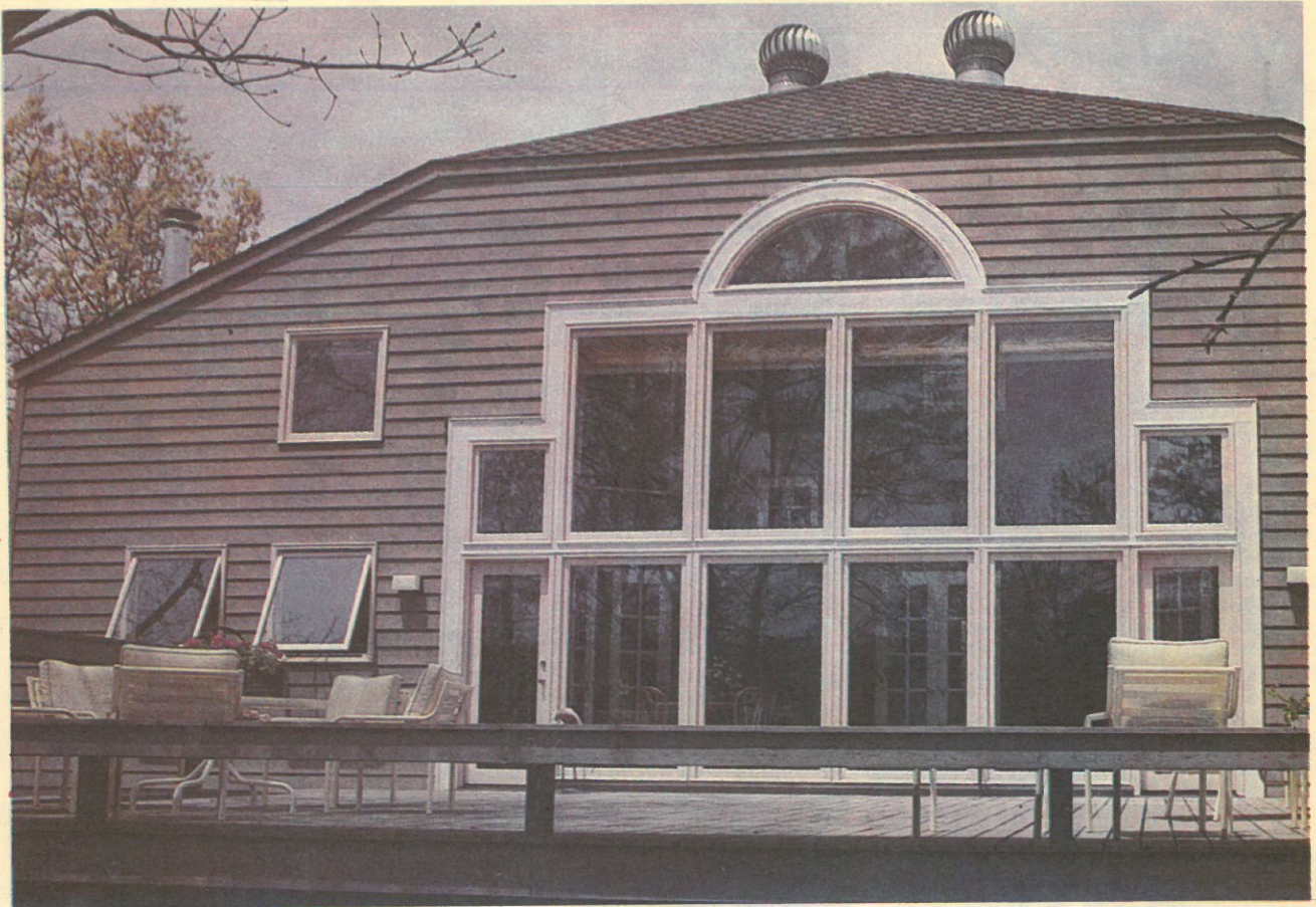
Jeffrey Milstein's passive solar house is built in a North-South direction. The south wall opens onto a sun space and has a huge window.
