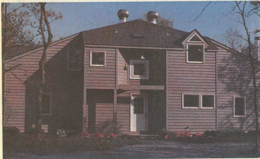
Jeffrey Milstein's passive solar house is built in a North-South direction. The south wall opens onto a sun space and has a huge window.
