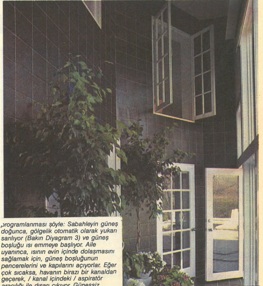
The sun space is covered with black-tile, which soaks up heat. This heat is distributed directly through the windows which the family opens in the morning.
