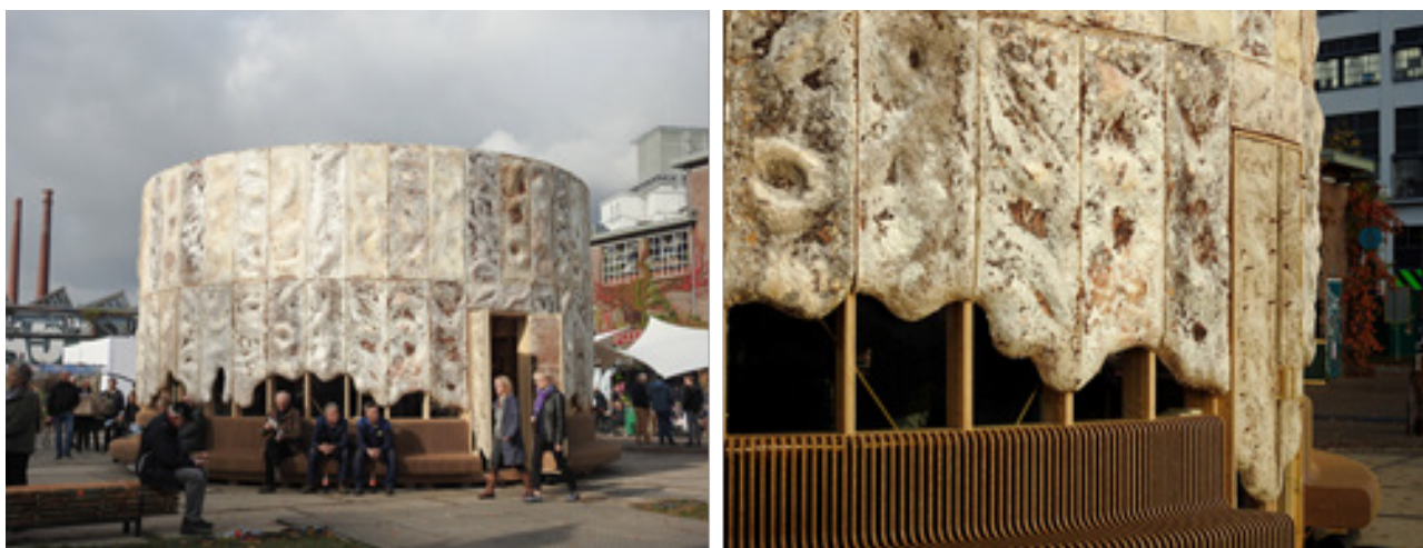
Figures 5-6: General view and close-up perspective of the Growing Pavilion (Mycelium Pavilion).
