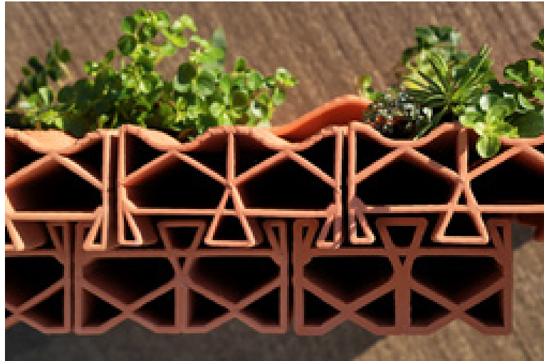
Figure 10: Partial view of Brick by Bit and the connection detail of the bricks. PA Editorial Team. (2024, July 30). Victoria Roznowski's "Brick By Bit" redefines clay bricks with 3D printing. Parametric Architecture. https://parametric-architecture.com/brick-by-bit-redefines-clay-bricks-with-3d-printing/
